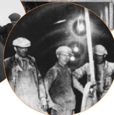
Clockwise from top: building Clatteringshaws Dam in 1933, Labourers lining Glenlee Tunnel, 1933, Workers in Glenlee Tunnel, 1933 Earlstoun workers
