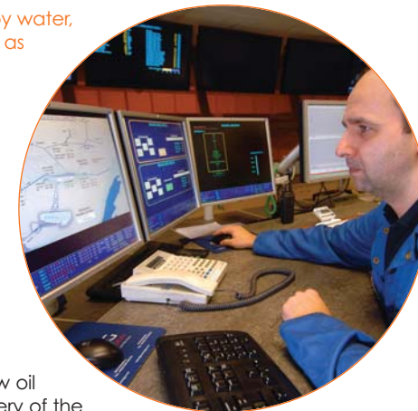
The control room
