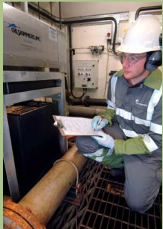
■ Checking the operation of oil skimmers at Cruachan
