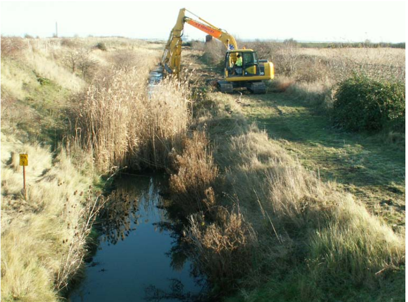
■ A mechanical digger clears vegetation from the Berry Wiggins drain to improve conditions for Water Voles at Damhead Creek
