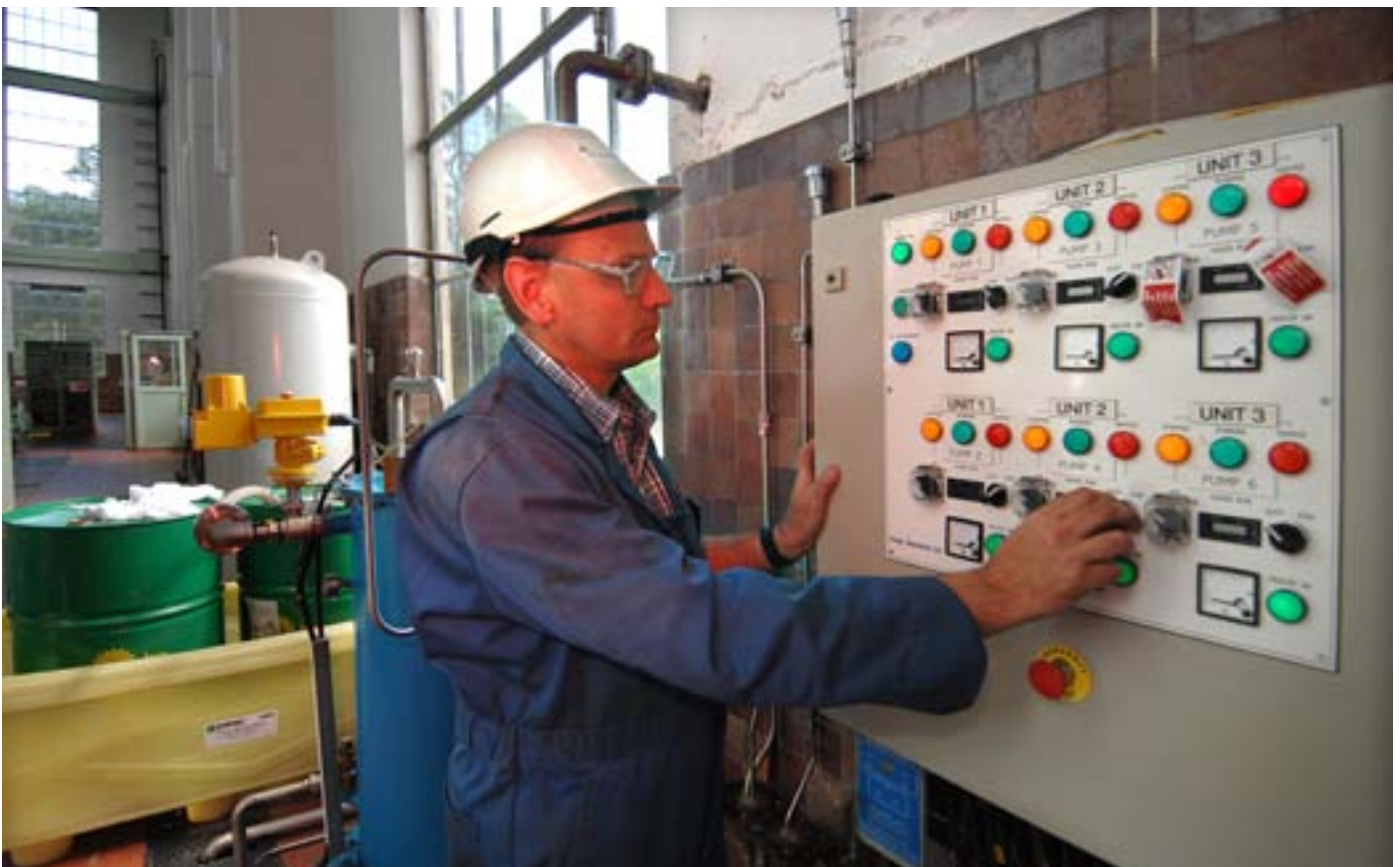
■ Glenlee Power Station Control Room – the nerve centre of the Galloway Hydro-electric Scheme
