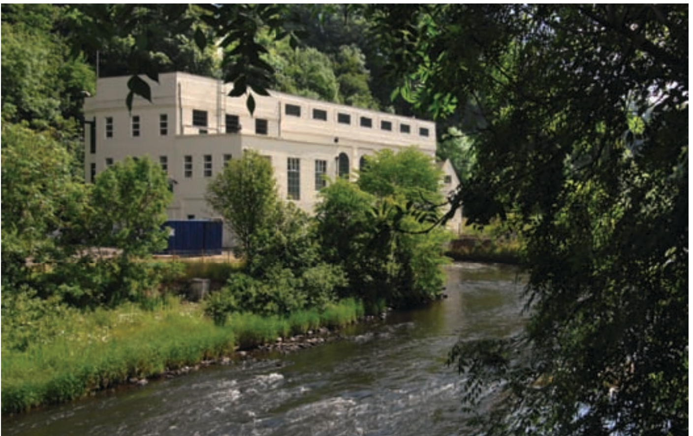
■ Bonnington Power Station, part of the Lanark Hydro-electric scheme, is a clean generator of sustainable electricity
