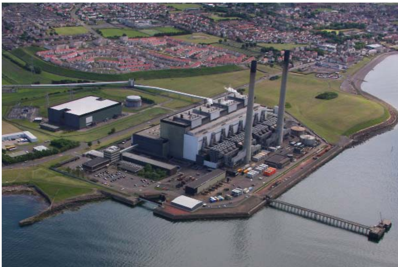
■ ScottishPower has submitted an application to replace Cockerzie's coal-fired station with a modern CCGT plant
