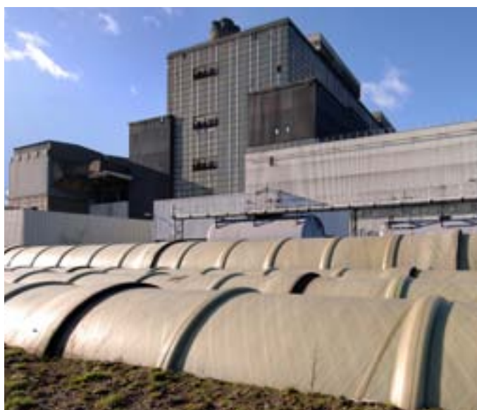
■ Construction work to retrofit Longannet Power Station with Flue Gas Desulphurisation SO 2 abatement system
