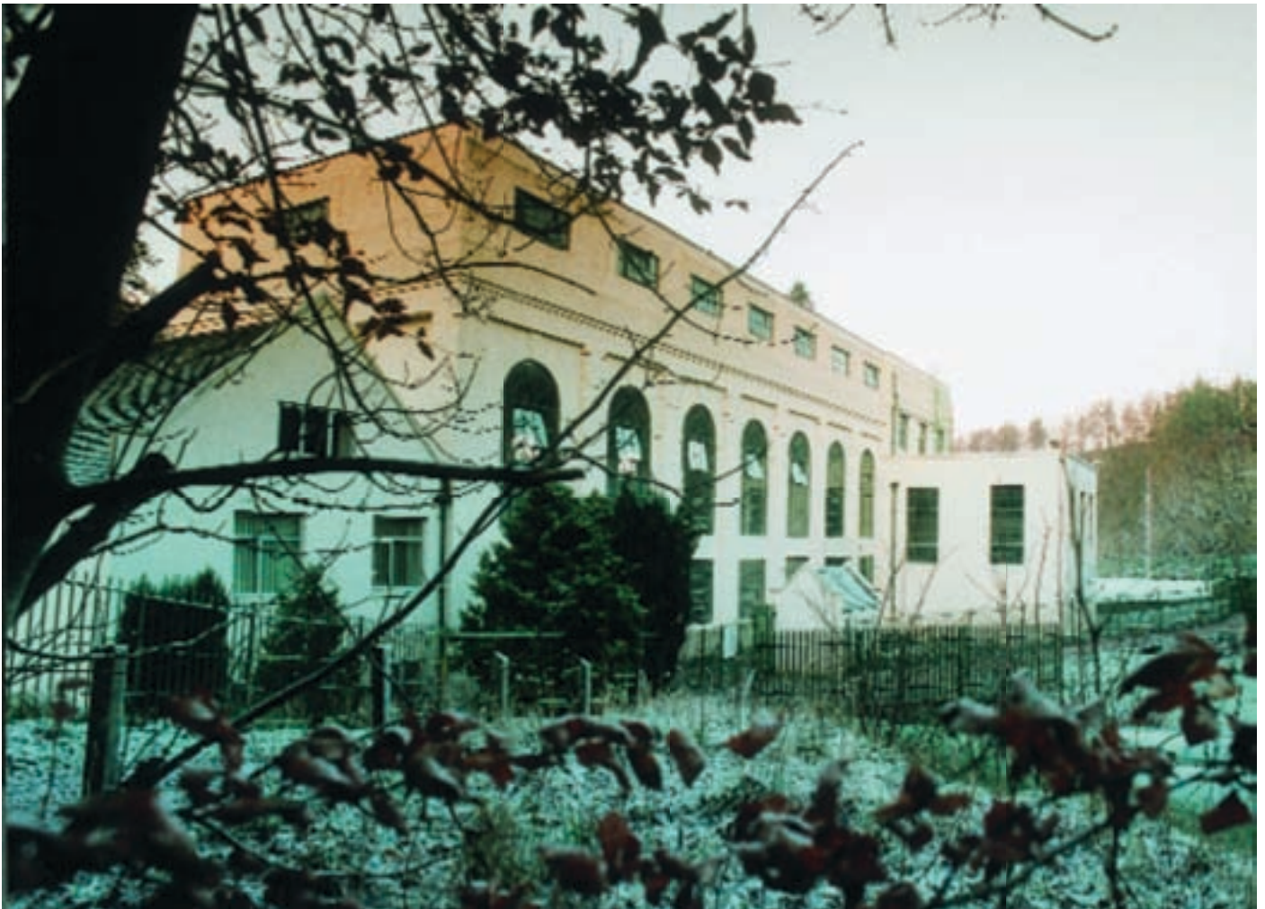
■ Bonnington Power Station at the Lanark Hydro-electric Scheme
