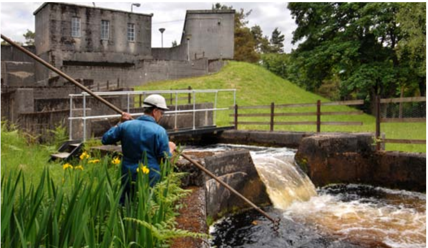
■ Maintaining the fish ladder at Earlstoun Power Station in the Galloway Hydro-electric scheme
