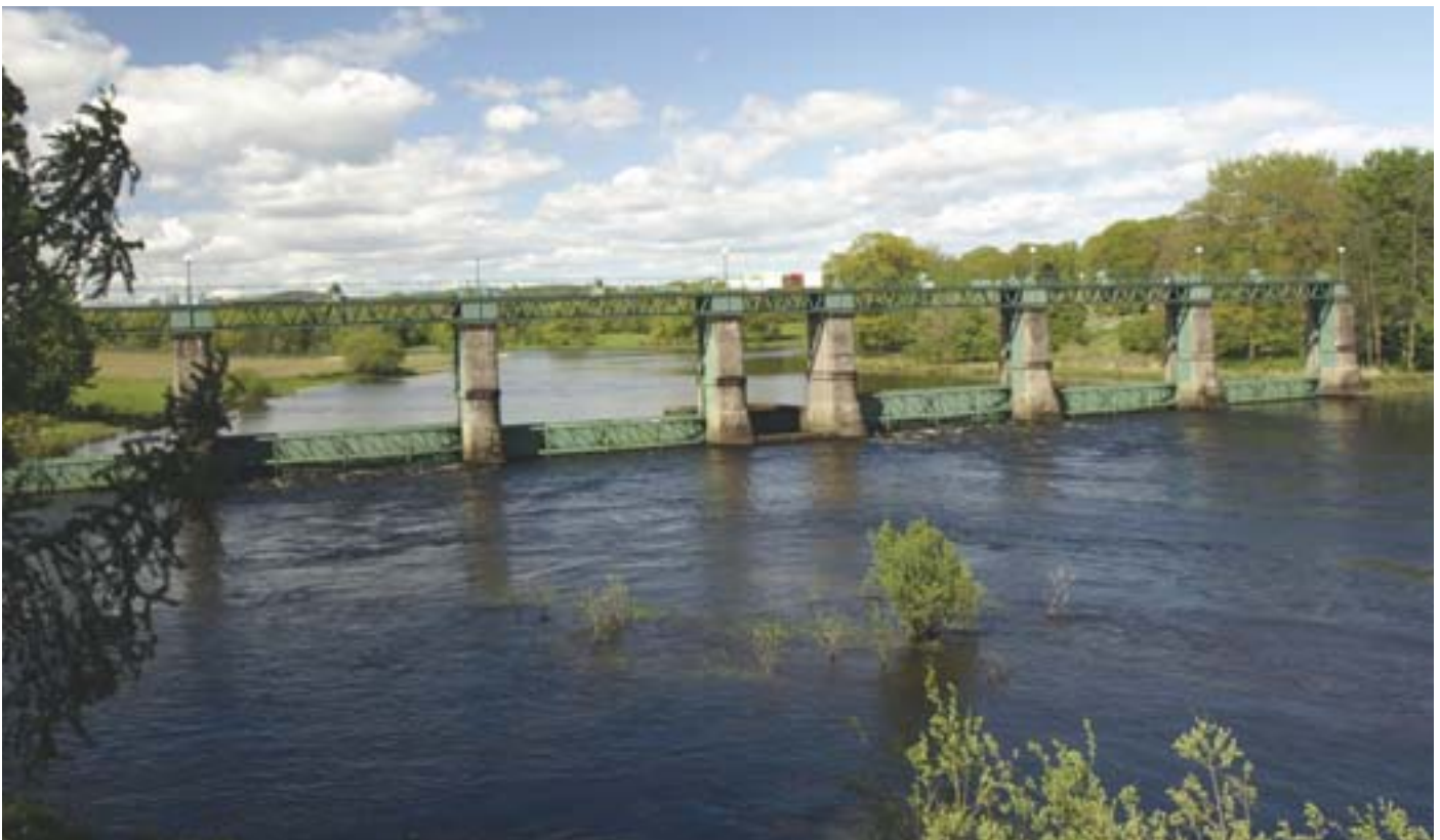
■ The Glenlochar Barrage, part of the Galloway Hydro-electric Scheme, helps to control water levels on Loch Ken
