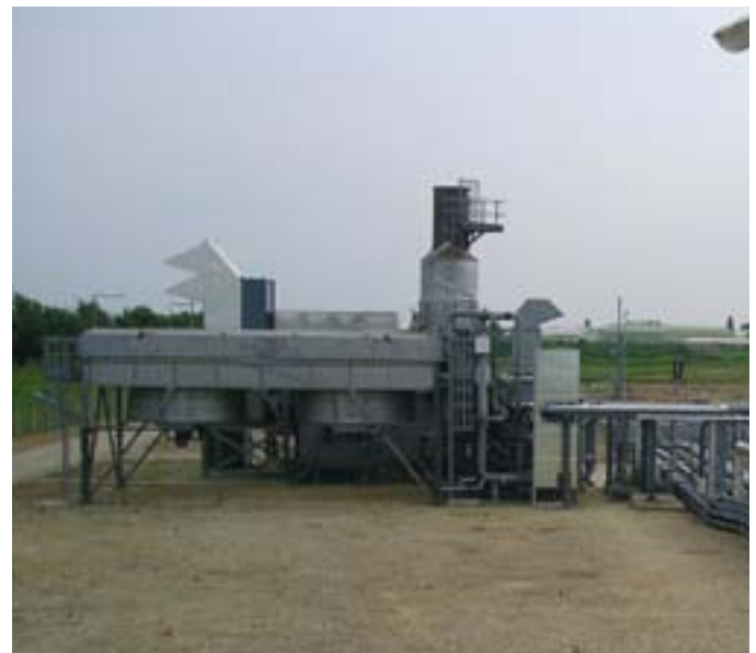
■ Hatfield Moor Gas Storage Facility, Yorkshire
