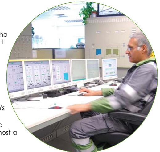
The control room
