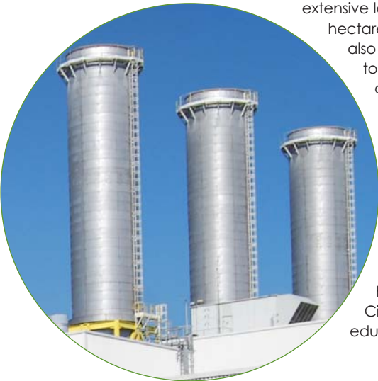
Rye House's distinctive triple stack
