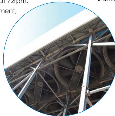
The air-cooled condenser
