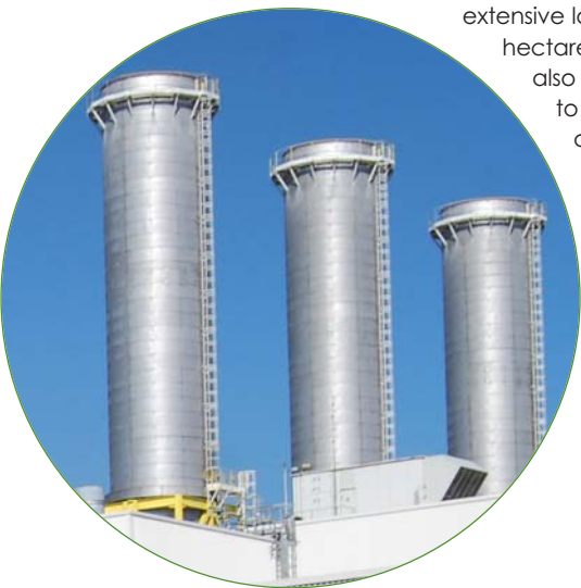
Rye House's distinctive triple stack
