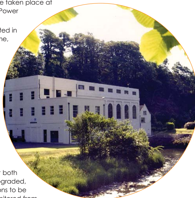
Stonebyres Power Station
