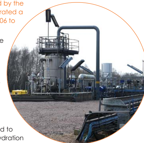
The well site
