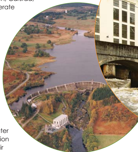
The 12 MW Carsfad power station has a 503m dam wall – the longest in the scheme
