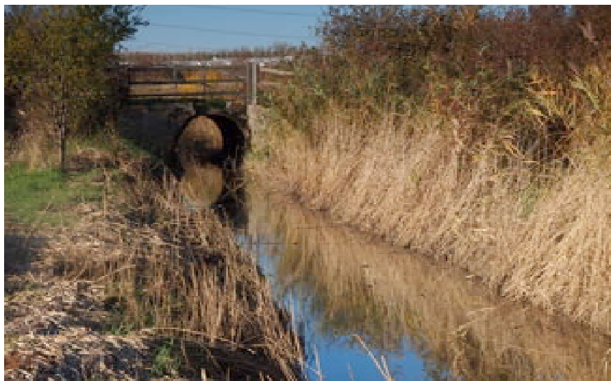
The Berry Wiggins Drain after ditch and vegetation clearance work was carried out in 2012
