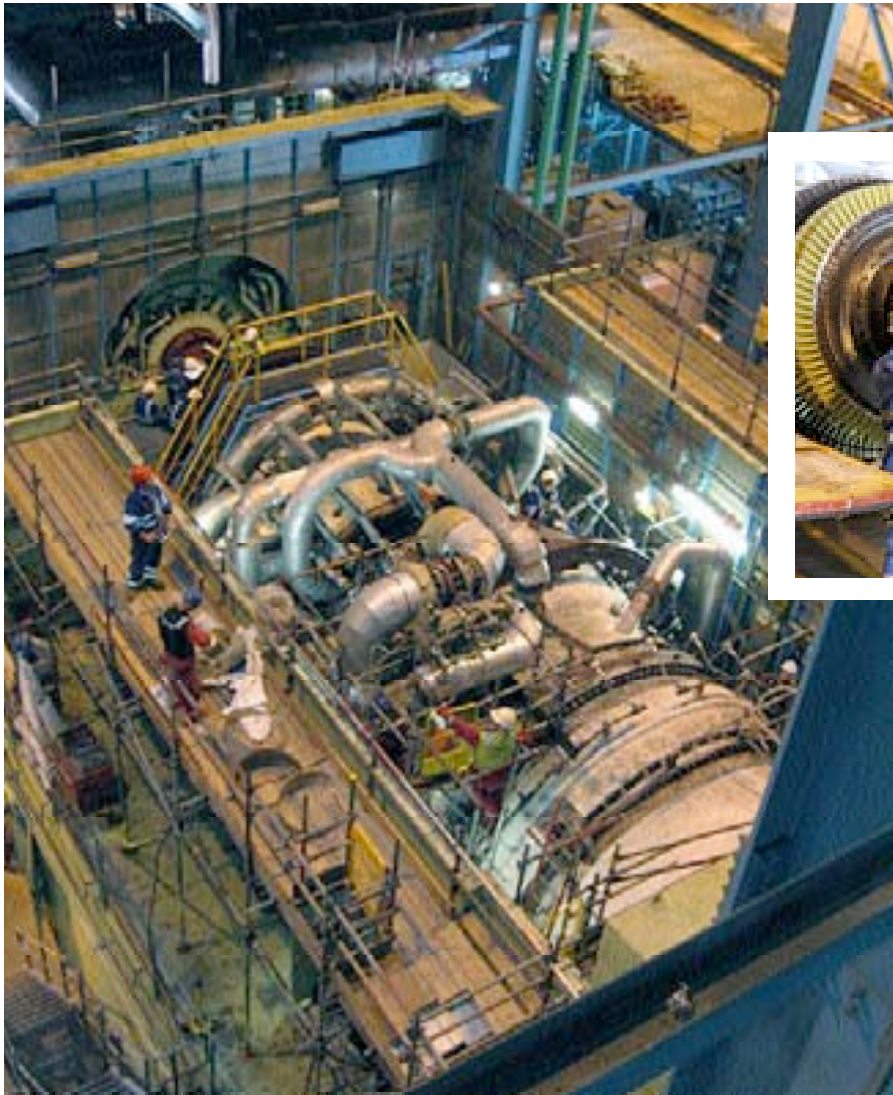
The gas turbine strip down is well underway and, right, GT compressor blades are exposed
