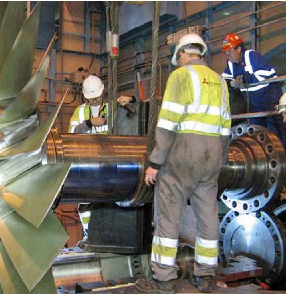
Gas turbine rotor blades are exposed during the 2012 outage that involved up to 200 contractors
