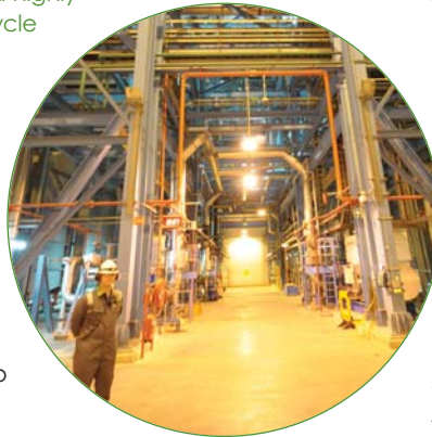
The plant runs continuously to meet demand
