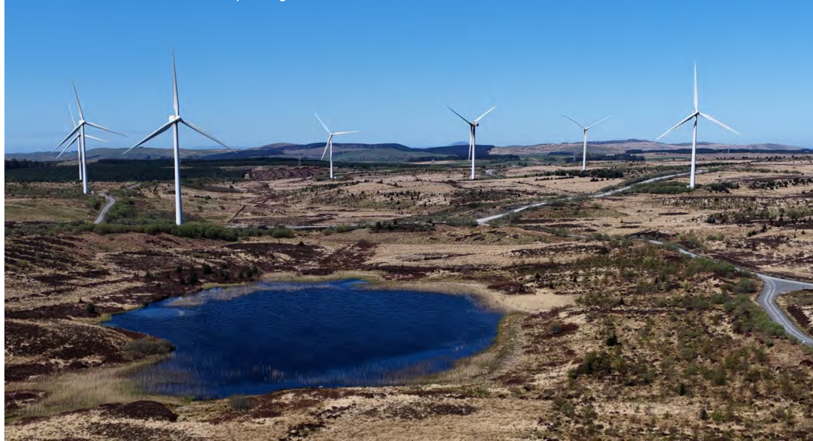
Peatland restoration and native tree planting at Mark Hill Windfarm
