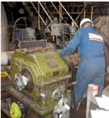
A specialist contractor carries out maintenance on Unit 2 feed pump during the major outage
