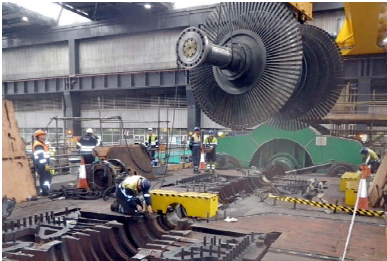
Station staff and contractors supervise as a massive turbine rotor is lifted into position on Unit 2 during the major outage that started in 2012 – see page 14
