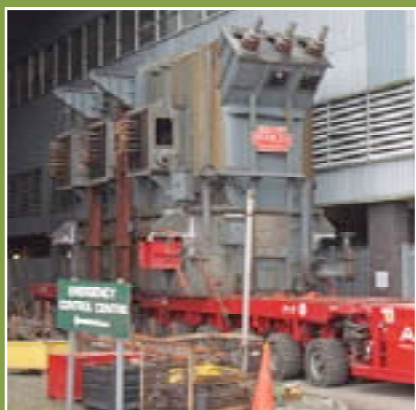
The new Smit generation transformer arrives at the station and, below left, the old unit is removed
