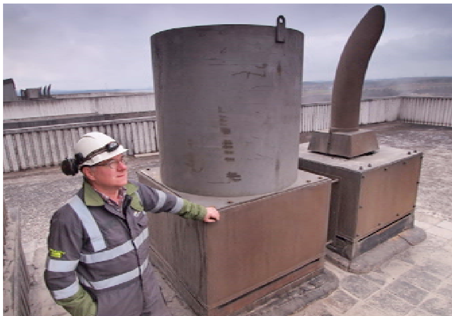
New safety valve silencers have been installed high up on the boiler roof to help control process noise
