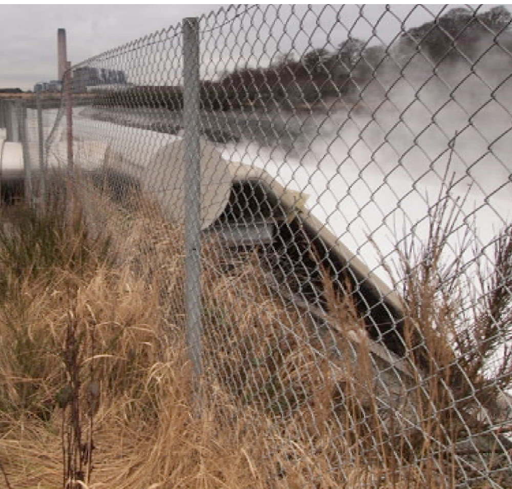
Cooling water returned to the discharge flume is monitored to ensure it meets permitted standards
