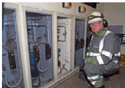
Inspection of the hydrazine dosing plant
