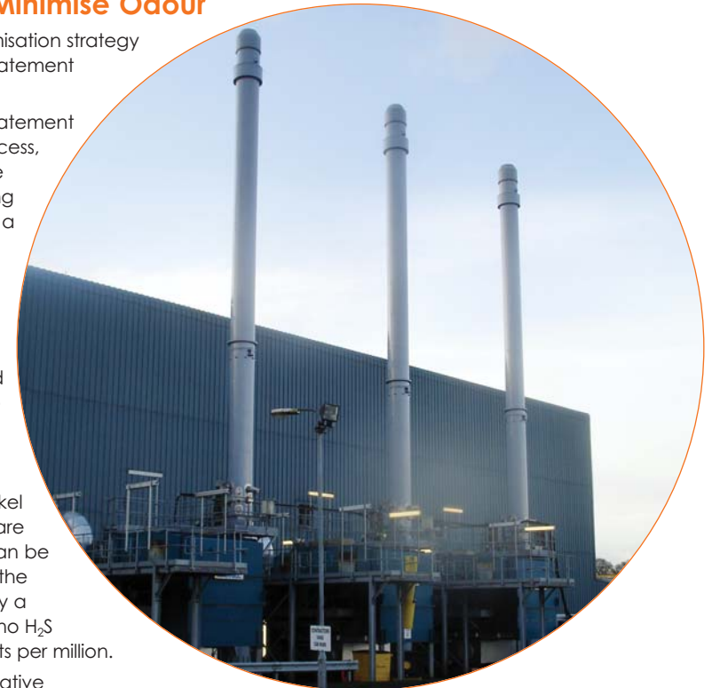
Daldowie's Regenerative Thermal Oxidisers (RTO) are on each of the stacks
