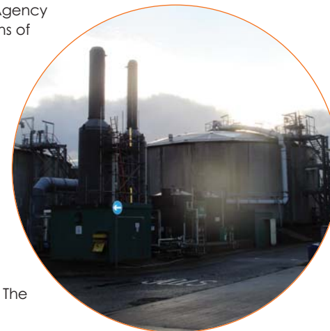
Daldowie uses sophisticated odour abatement technologies
