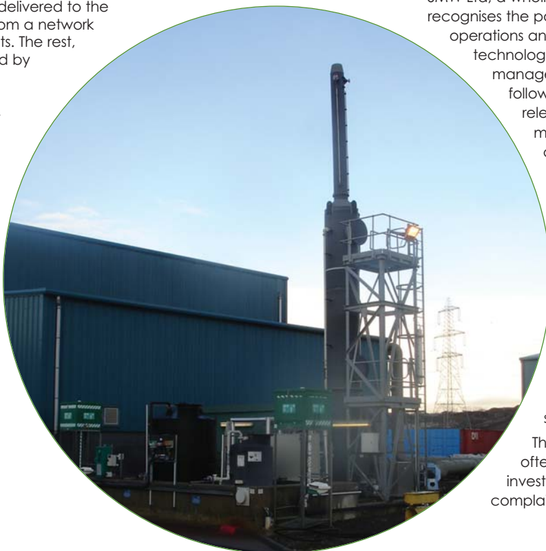
Odorous air from the Lamella settling tanks is drawn off and passed through a scrubbing mixture
