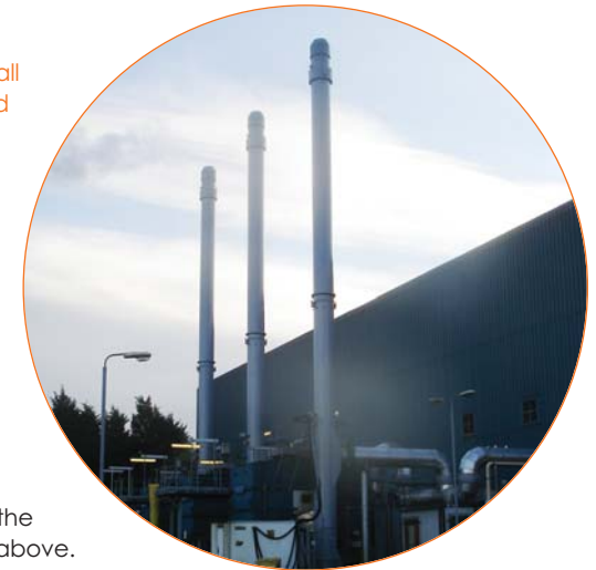
Daldowie has Regenerative Thermal Oxidisers (RTO) on each of its three exhaust stacks to abate odour
